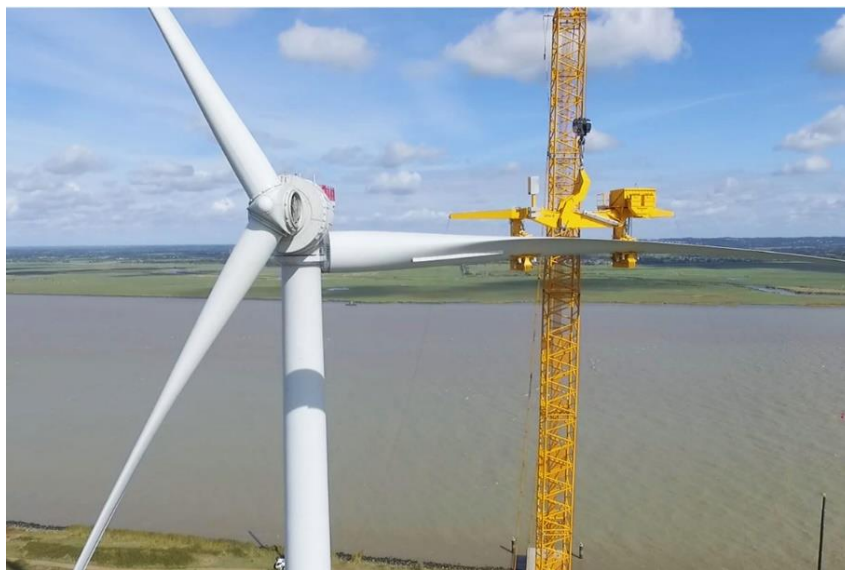
Figure 7: Blade Lifting tool for installation
