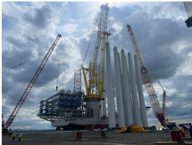
Figure 3: Tower load-out
